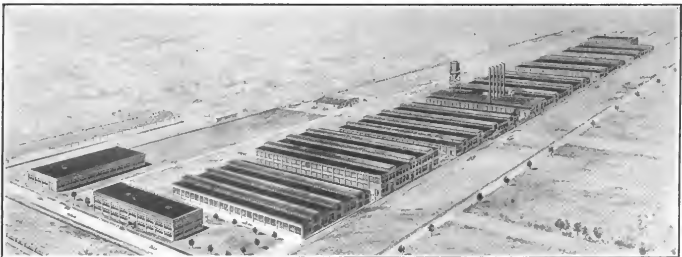
❶ The new plant of the Willard Storage Battery Co., Cleveland, O., when completed, will contain 6 acres of floorspace, leaving ample land for further expansion. Ten buildings will comprise the plant. All buildings will be of brick, of the latest approved and most up-to-date construction and equipped with sprinkler system throughout. The various buildings will be entirely separate, sufficiently isolated
